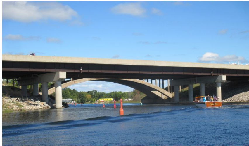
Return trip under Hwy 400 bridges, just before the lock.
